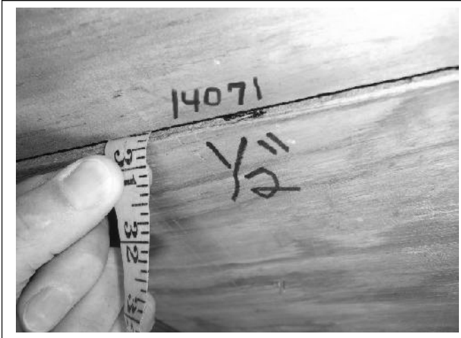
ROOF DECK THICKNESS – ½ inch plywood
