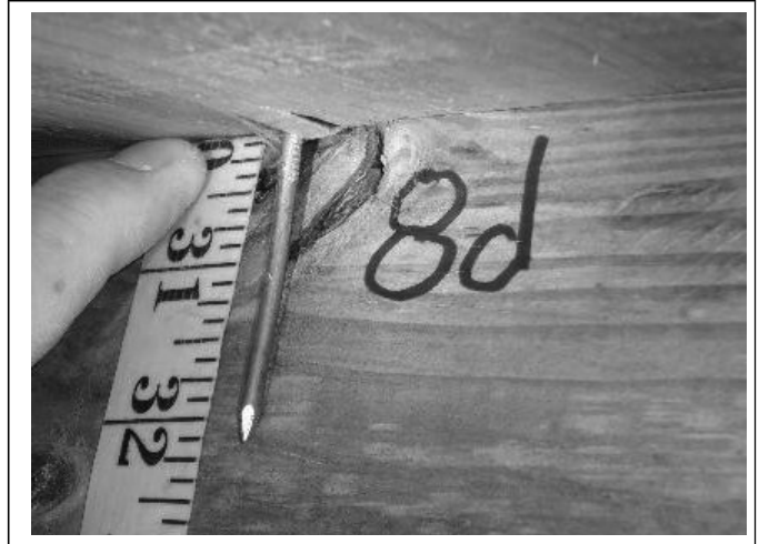
ROOF DECK ATTACHMENT – 8d nail
