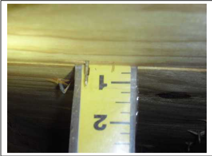
ROOF DECK THICKNESS
