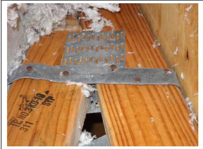
ROOF TO WALL ATTACHMENT
