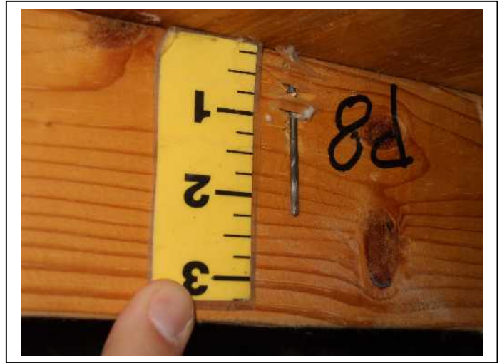
ROOF DECK ATTACHMENT
