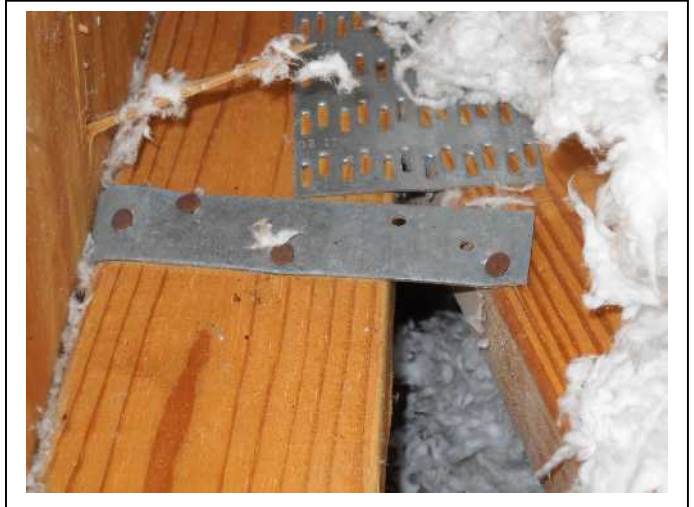
ROOF TO WALL ATTACHMENT
