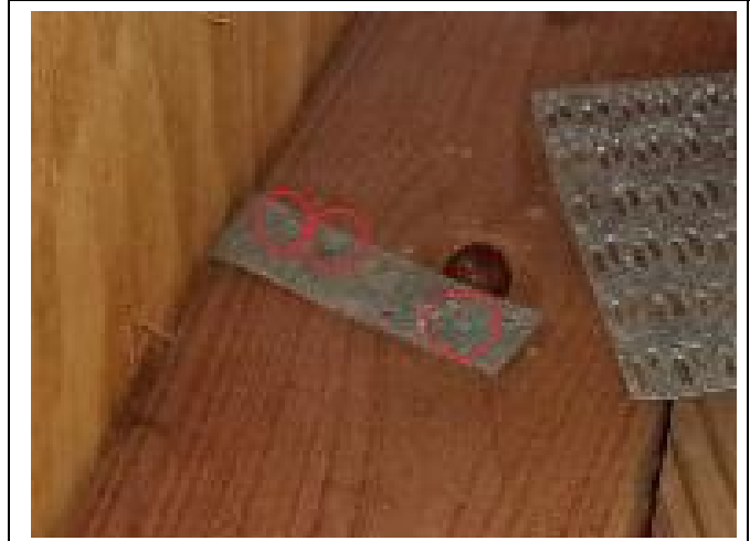
ROOF TO WALL ATTACHMENT – Properly installed Single Wraps
